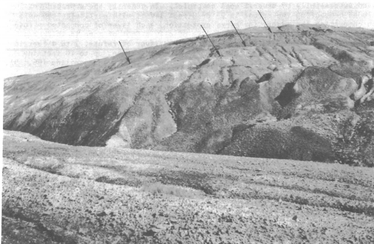
FIGURE 4. - Coal Refuse Sealing at the Cadogan Mine. Refuse layers can be identified by parallel line effect in the pile, as indicated by arrows.
