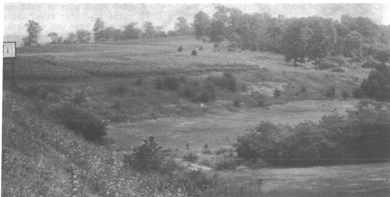
FIGURE 7. - Land Restoration to Contour at Abandoned Coal-Stripping Operation Near Greensburg, Pa. Restored land planted to corn. Previous highwall follows tree line in background.
